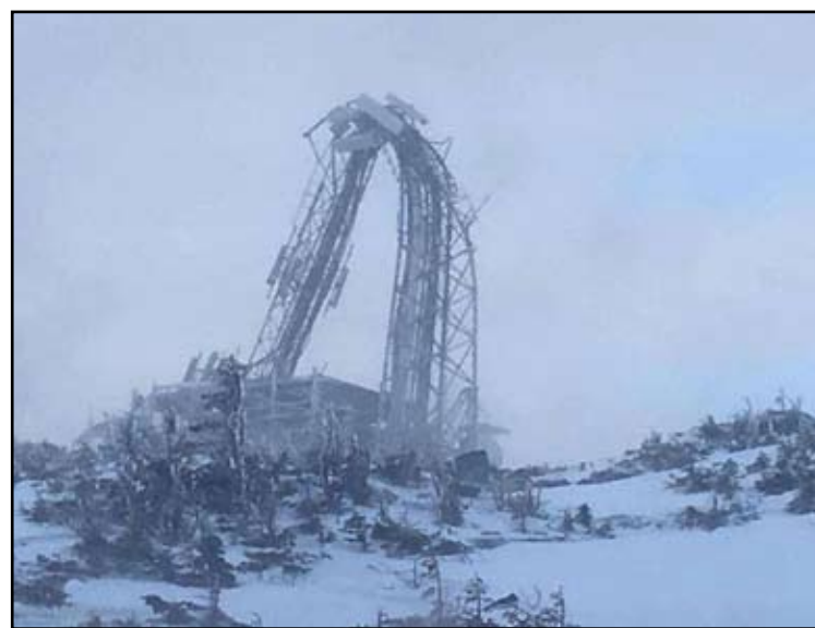
A communications tower on Sugarloaf mountain was no match for the 100 mph gusts recently, as shown in this image originally taken by winch operator Trevor Dakers.
